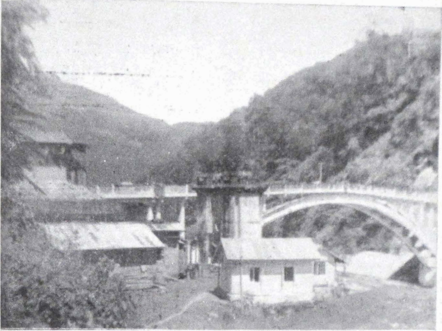
ON WAY TO GANGTOK—TEESTA BRIDGE.
